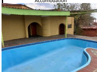
Empty swimming pool
